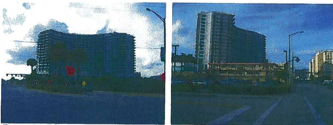
Figures 3.4-3.5 – Oceanside Plaza of Pompano Beach Condominiums
