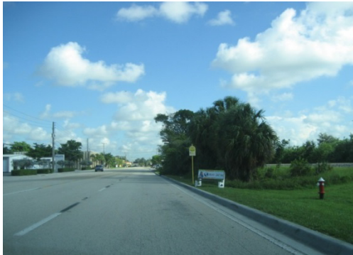
Bus stop on northbound Dixie Highway north of Cypress Creek Canal without sidewalk connections
