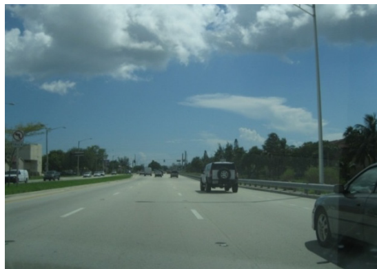
Six-lane and four-lane segments of Atlantic Boulevard within Pompano Beach
