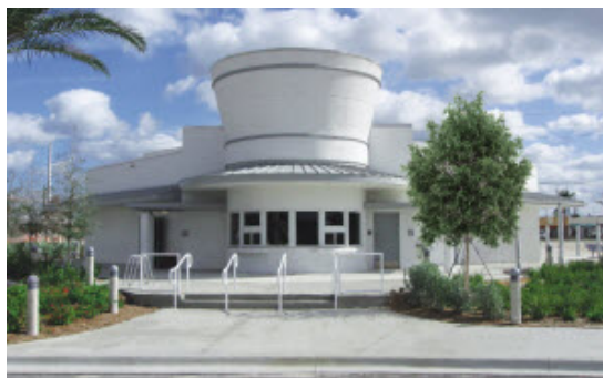
New Bus Transfer Facility near Dixie Highway and Dr. Martin Luther King Boulevard
