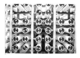
**Project Description:** This ongoing project consists of replacing the membrane elements (filters) when needed. The membrane elements are used to purify water to make it potable and requires replacement every 5 years. All filters were replaced in FY 2016. Funding will be budgeted over a multi-year period to provide for full replacement.
