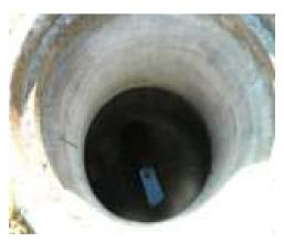
**Project Description:** This project involves the rehabilitation of deteriorated brick manholes located throughout the City. Rehabilitation consists of covering the interior surfaces with an adhesive, non-permeable material. 58 manholes have already been relined in FY 2015. Citywide there are 4,400 manholes.
