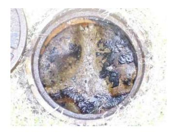
**Project Description:** This project involves the rehabilitation of deteriorated brick manholes located throughout the City. Rehabilitation consists of covering the interior surfaces with an adhesive, non-permeable material. Citywide there are 4,400 manholes.
