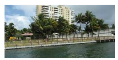
**Project Description:** The City is responsible for the maintenance of seawalls along City-owned property; there is approximately 2,000 linear feet of seawall along various canals and waterways. Maintenance can include rebuilding portions, grouting leaks and total reconstruction.
