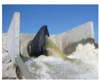
**Project Description:** This project is to install check valves on tidal outfalls. The valve will prevent backflow of tide onto streets during extreme high tides, when tidal waters are higher than the roadway.
