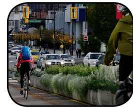
4 10-14 foot widened landscape medians
