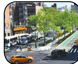
4 10-14 foot widened landscape medians
