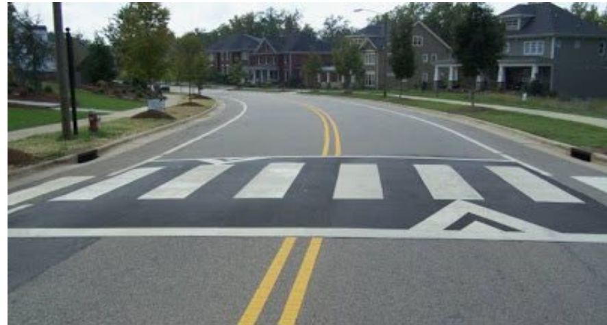
Raised Crosswalk (Speed Table)
