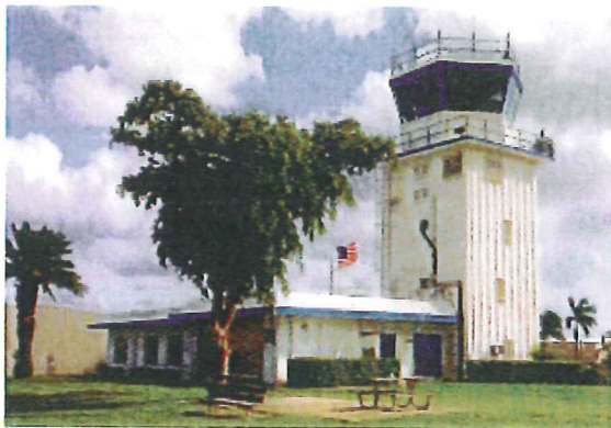
Figure 3.2: Administration Building and Control Tower
